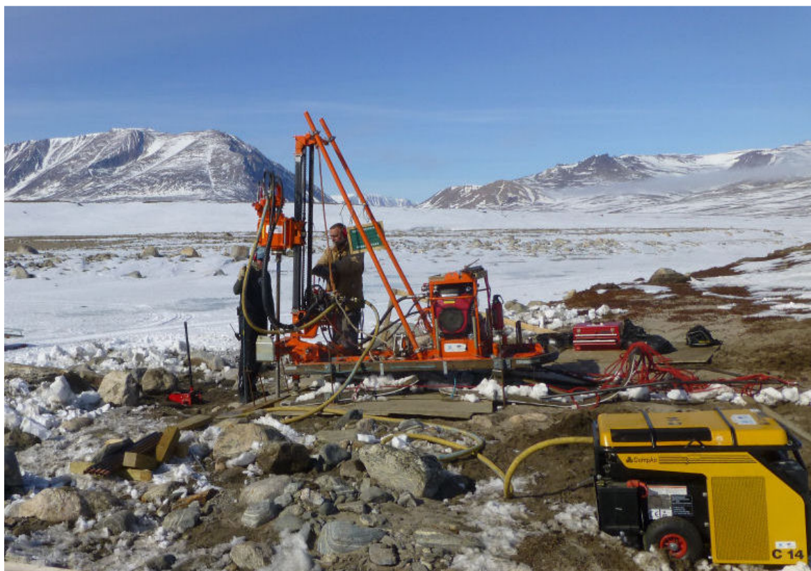
Drilling holes for the foundation of the new bridge at the Zackenberg May 2013. Photo: Mikkel Tamstorf.
