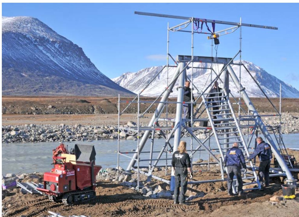
Figure 6.45 The bridge was put together on-site by a crew of seven people using mainly hand power. Photo: Jørgen Skafte.
