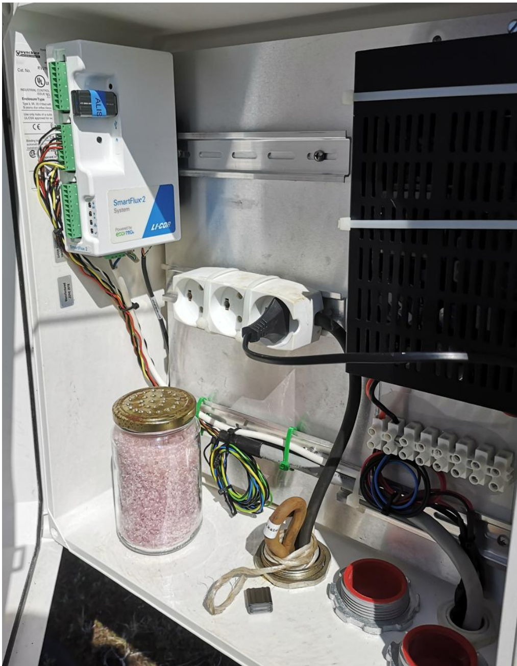
Figure 3.3. Inside the EddyFlux box the SmartFlux2 module is found (#7 in Figure 3.2).
