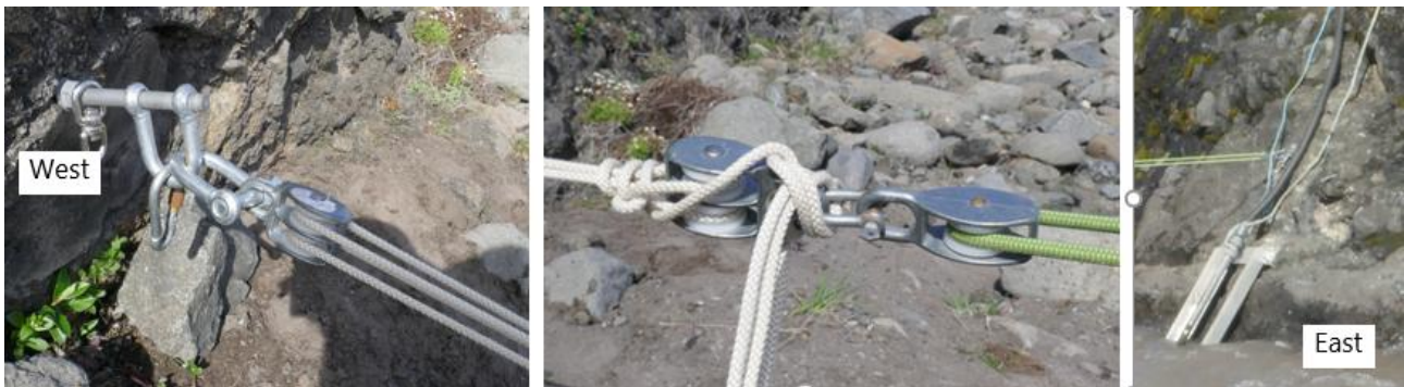
Figure 6.11. The rope is running across the river in a loop. The white rope near the wall makes it easier to adjust and tighten the rope loop.
