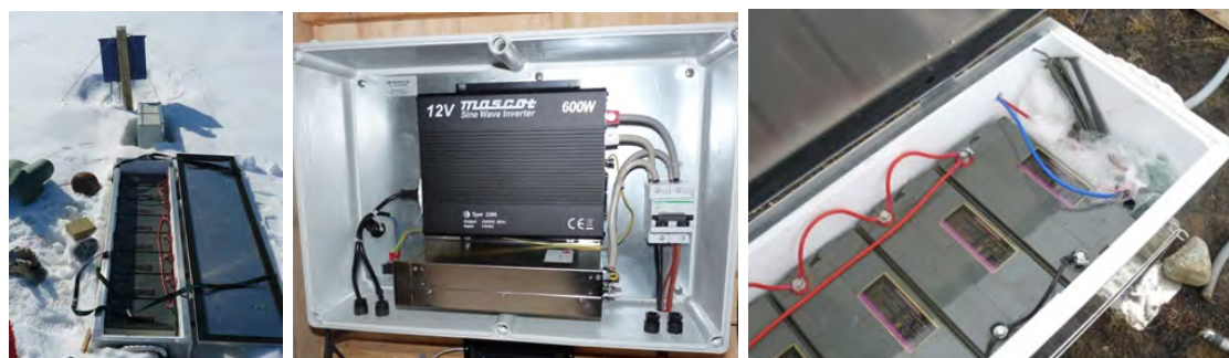
Figure 75: The battery box (left). A look into the transformer box, inside the hut (mid). Power cable from the instrument box enters the battery box in the southern end –the red and blue cable are connected to plus and minus on the last battery in the row.
