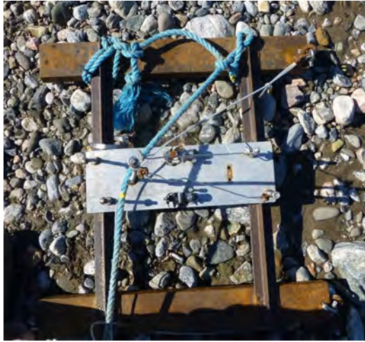
Figure 49: Metal frame for installation of pressure transducers
