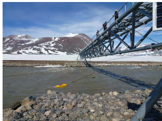
Figure 54: Discharge measurements are performed along the hoist trolley. Qliner is attached to the steel wire.
