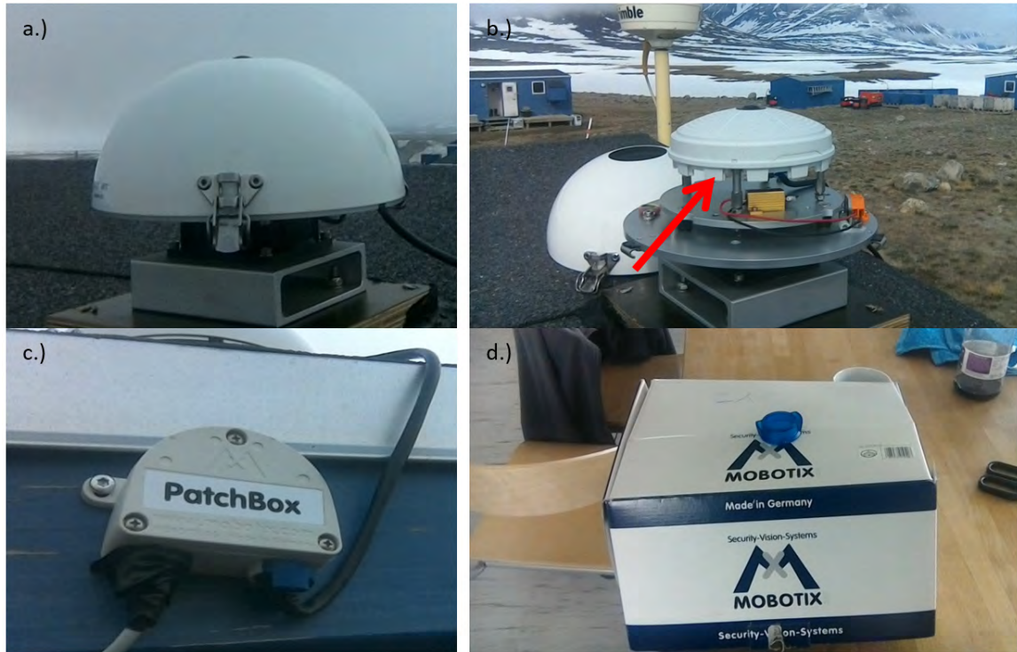
Figure 40: Sky camera operational in ventilation unit (a). To uninstall the camera, remove the white protection shield, lift the camera from the base plate (b) and unplug the black Ethernet cable from the Patch Box (c). Store the camera over winter in the original box with the blue protection cover over the lens (d).
