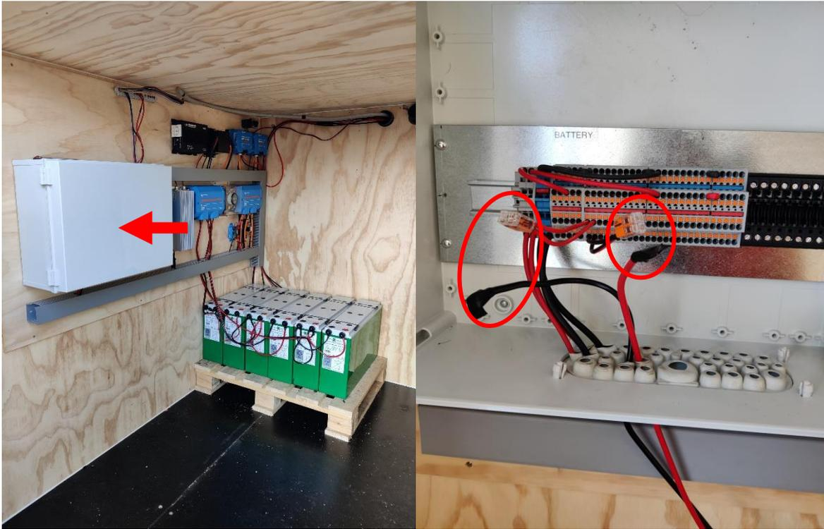
**Figure 20** Power setup at the Heath location. To disconnect Eddy Heath from power, disconnect the cables in the samlemuffe in the grey box.
