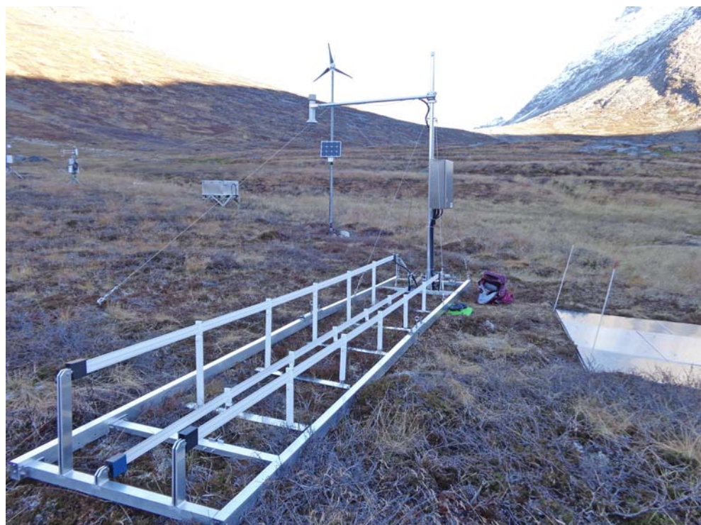
Figure 3.1 A new Snow Pack Analyzing System was installed at the heath site in August 2013. In the background the new wind generator and solar panel for the power supply can be seen.
