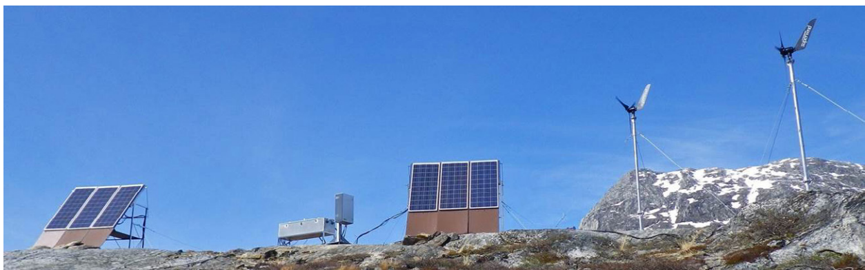
Figure 3.9 In order to minimize the number of gaps in the time series from the climate station and the two flux stations at the Fen location, two 350W wind generators and four new 100Ah batteries were added to the existing power supply of six 110W solar panels and 8 100Ah batteries.
